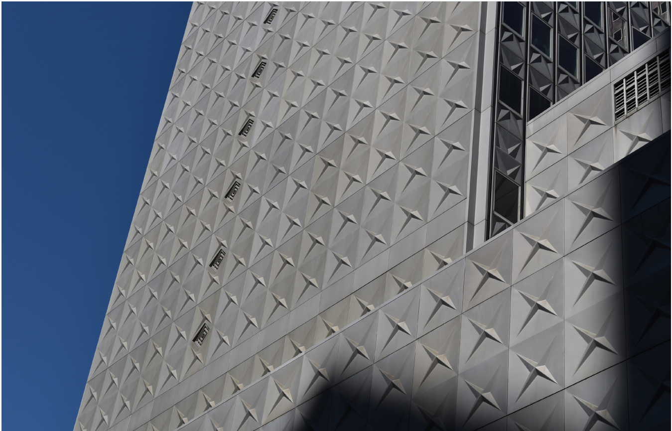
Figure 3. The Republic National Bank Building, Dallas, Texas (1954). Image Credit: Worth B. Chollar.
